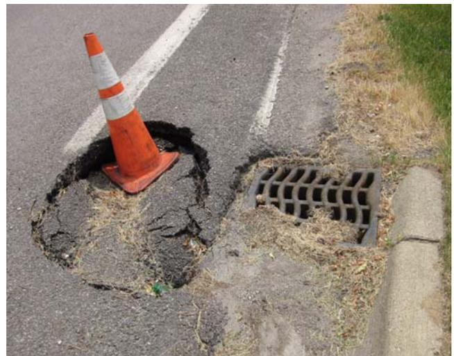
Figure 5. Damaged drainage system
