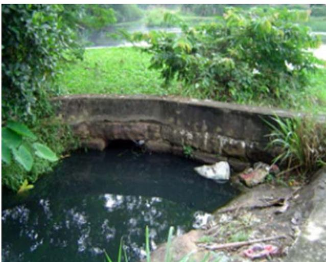
Figure 4. Blocked drainage system
